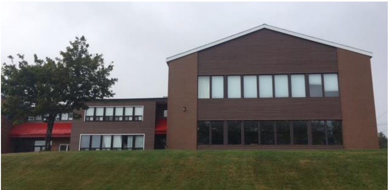
Photo 2. Close up of newer addition exterior.
