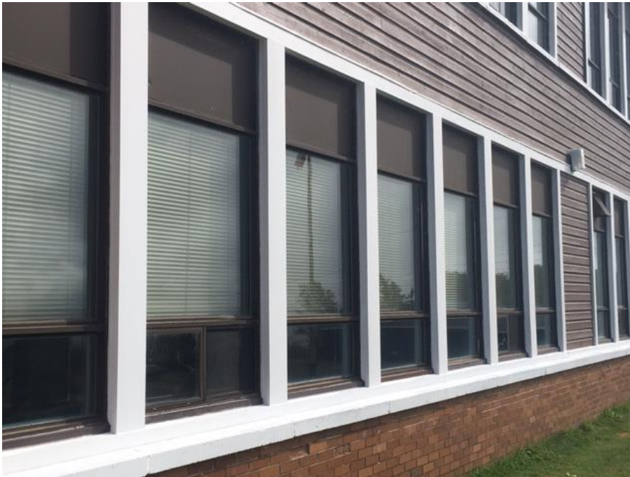
Photo 4. Windows on west side of entrance showing sill replacement.
