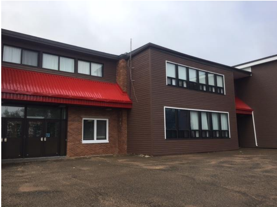
Photo 5. Close up of entrances to original and newer addition sections of the building.
